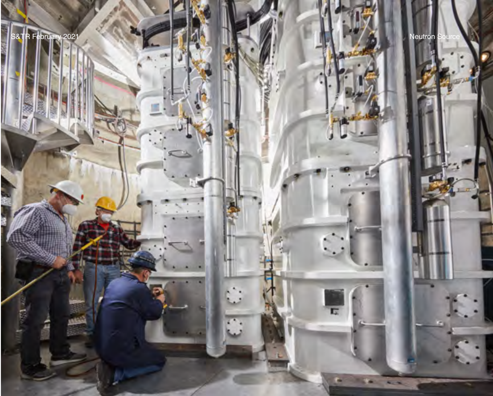
Capacitor towers providing 2 megajoules of stored energy fill the floor below the chamber where the plasma and neutrons are produced. (Photo by Garry McLeod.)
